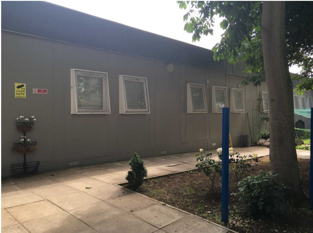
Photograph showing existing building
